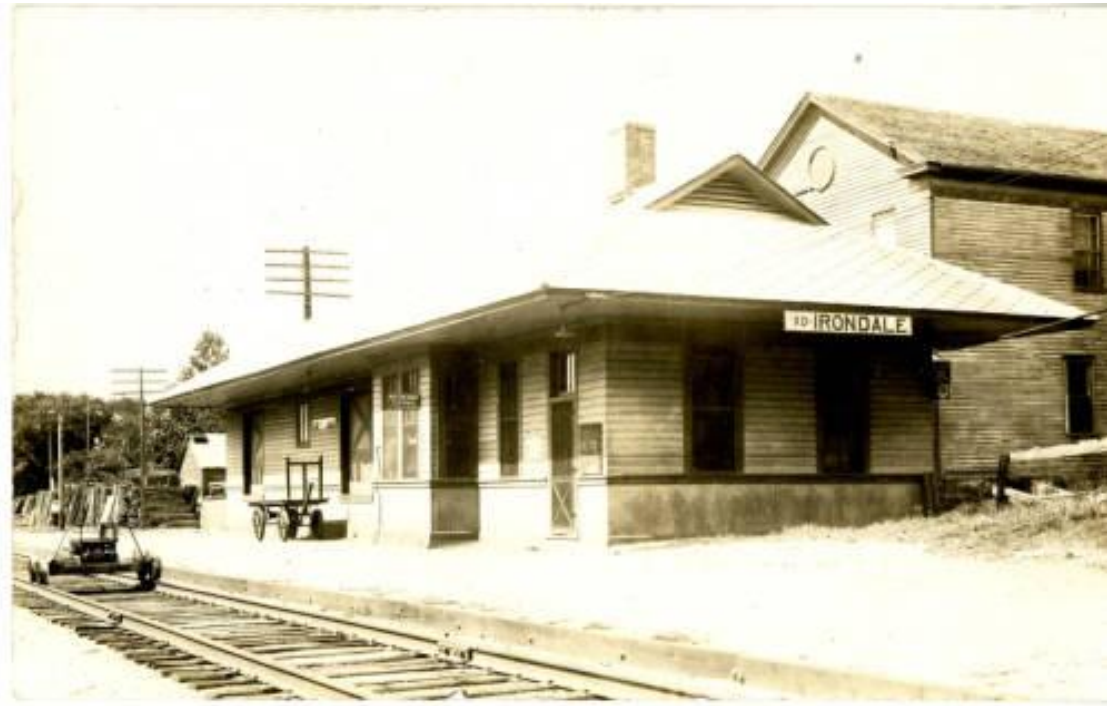
Irondale, Missouri Railroad Station (1930)
