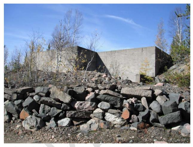
Photo 2: Foundations of the former Bidgood Kirkland Gold Mines Ltd. 125 ton per day mill.
