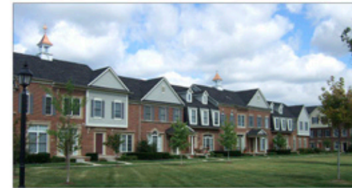
UNIFORM SITE LIGHTING ADD DORMERS, CUPOLAS, GABLES ADD INDIVIDUAL PORCH DETAILS VARY RAILING DETAILS VARY DOOR DETAILS
