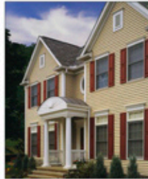
HORIZONTAL SIDING PORCH (PHASE II)
