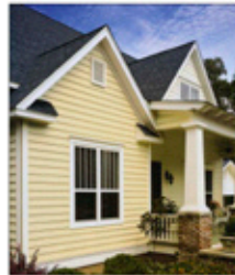
BEADED SIDING PORCH (PHASE II)
