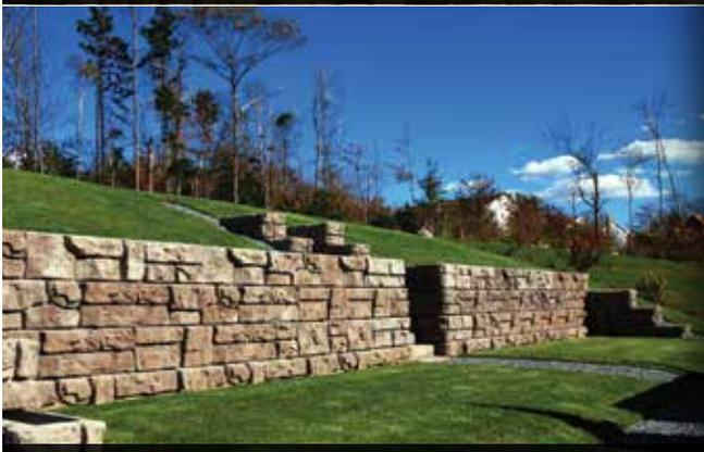
**Gravity** - Massive, one-ton Redi-Rock blocks rely on gravity to hold back slopes in many different applications, including this Ledge-stone wall. Even taller reinforced walls are possible; visit [www.redi-rock.com](http://www.redi-rock.com) for more details.
