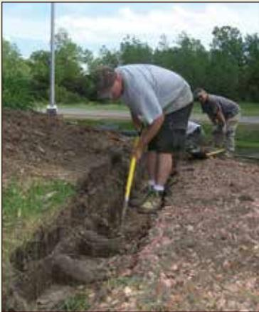
Excavate a trench the length of the wall, 24 inches wide and deep enough to accommodate 6 inches of crushed rock base material and the embedded courses. If your wall requires geogrid soil reinforcement, the area behind the wall where geogrid is placed also must be excavated (see Step 5).
