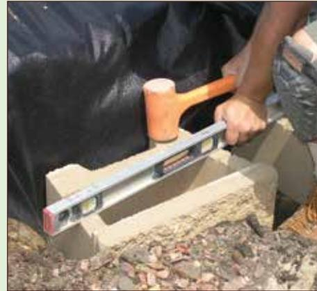
Anchor VERSA-Green CG behind bottom units with 6 inches of CG placed horizontally on top of the leveling pad. Then wrap CG vertically behind embedded units. Place soil backfill behind embedded units and VERSA-Green CG. Also replace and compact over-excavated soil in front of the units. Remember—the backfill behind and in front of embedded units should consist of soil. Do not use drainage aggregate.
