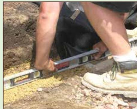
Using a 4-foot level, level units front-to-back and side-to-side with adjacent units. Tap high points with a mallet or hand tamper until level. After positioning the base course, fill the cores of all completely buried units with the same crushed gravel, as was used for the leveling pad. Partially exposed units should be filled with planting medium to promote plant growth.
