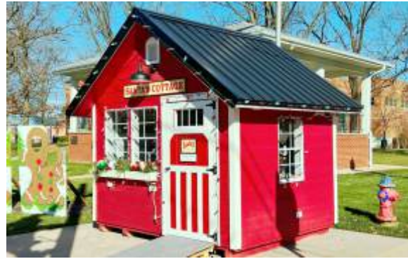
Painted Victorian with three windows and transom in door
