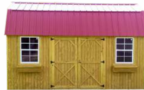
Wood siding with metal roof
