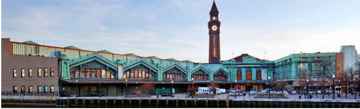
Figure 22: After Superstorm Sandy, the city of Hoboken, New Jersey worked with financial experts to develop a multi-purpose solution that includes green infrastructure, open space, parking capacity, and sub-surface stormwater protection. Source: Re:Focus website and Re:Invest: A Roadmap for Resilience, used with permission
