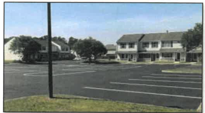
Thanks to the Board for scheduling the Milling and Paving of our Streets in April 2023. What a difference this has made in the overall appearance of the neighborhood!
