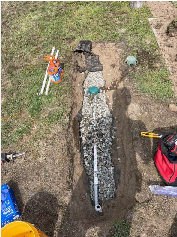
Bottom facing orifice appears to have a missing orifice shield. Orifice shield has been placed.
