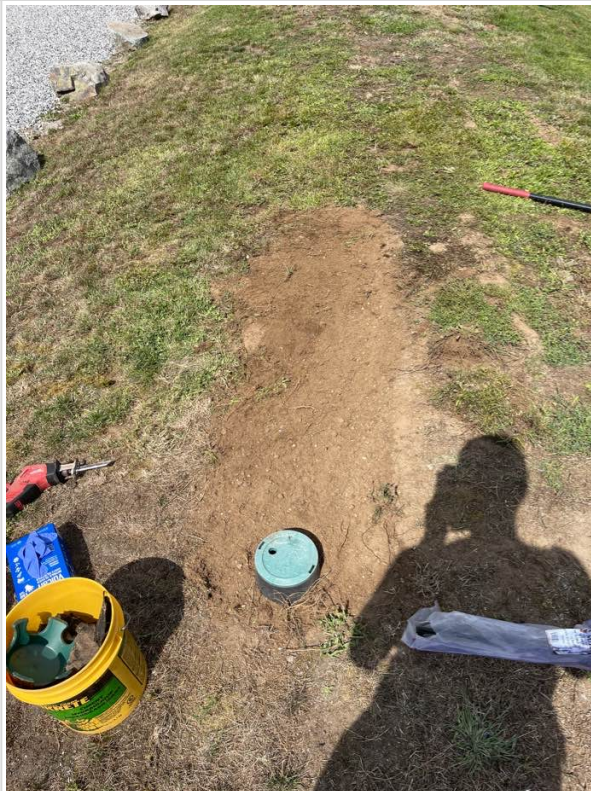
Lateral after backfill.
