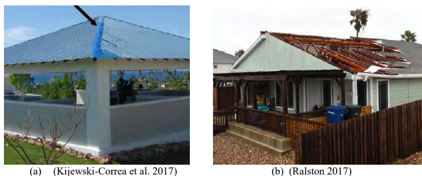
Figure 1: Example photos of (a) minor roof damage and (b) major roof damage provided to assist respondents
