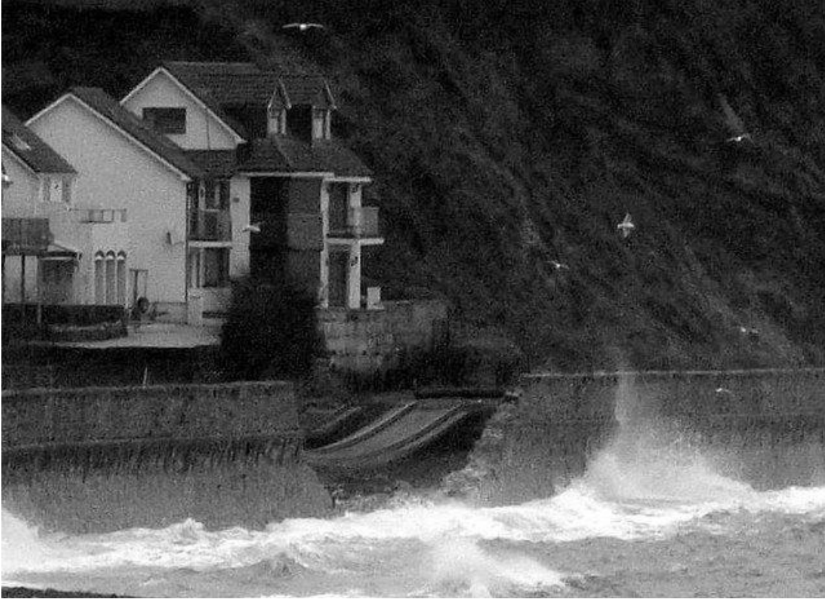
Figure 1– Collapsed sea wall in Dawlish, UK (Copyright Derek Harper and licensed for reuse under this Creative Commons Licence)
