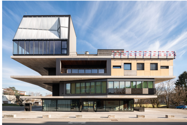
Figure 1.1: NEST with DFAB HOUSE (top left). Photo: Roman Keller
