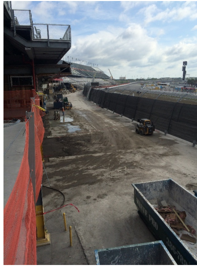
Figure 1: Daytona Speedway - showing partial demolition of the 'frontstretch' seating.
