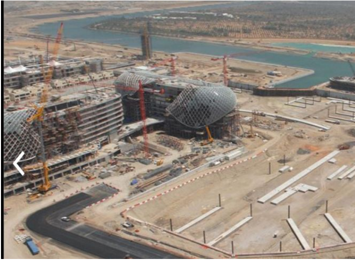
Figure 2: Yas Marina F1 motor racing construction site – Yas hotel and its' grid shell
