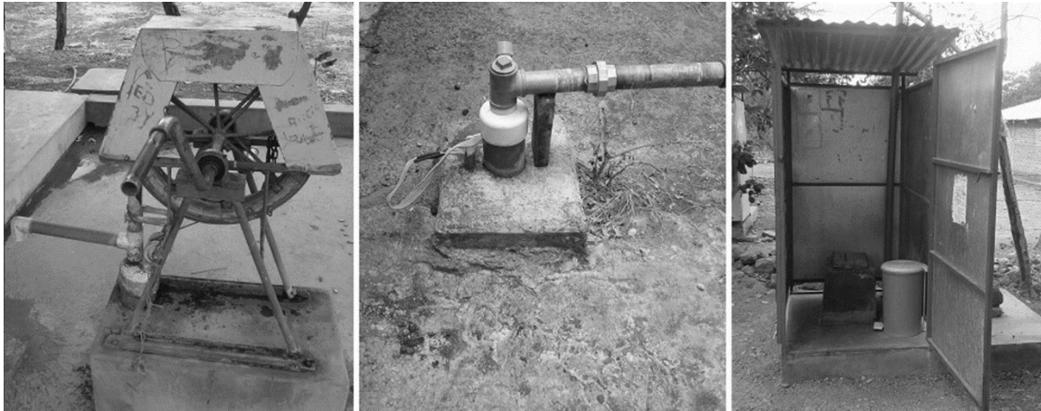
Figure 1. The three primary WatSan technologies in Darío. Rope and electric pumped wells (left and middle, respectively), ventilated improved pit latrine (right).
