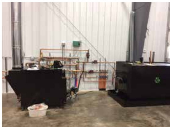
2 Waste Oil Boilers at Kuhns Equipment ~ Arthur, IL
