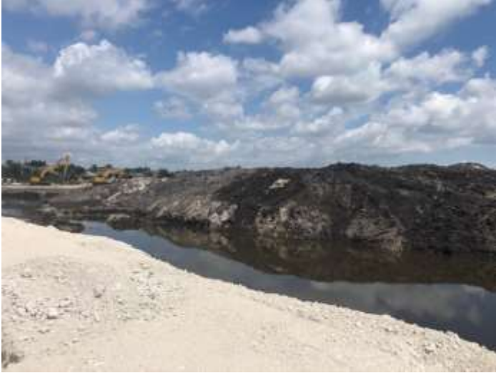
EXCAVATION OUTSIDE LOT 26 (SUNIL's neighbor) on March 20, 2021
