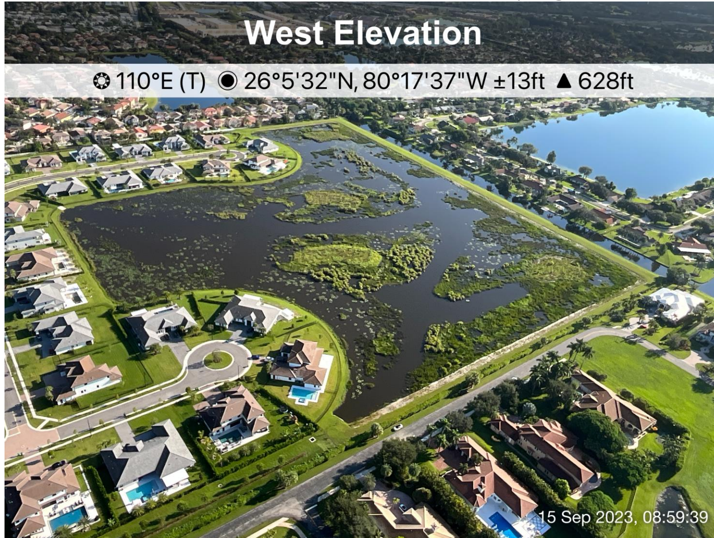
Inspection photo from South Florida Water Management District (SFWMD), Sep 15, 2023
