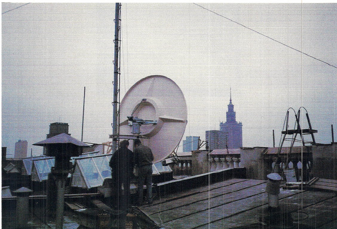
OrionNet and Vesatel engineers install VSAT on roof of Polish PTT at pl. Malachowskiego in Warsaw. The building in the background is the Palace of Culture and Science.
