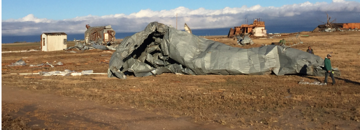
Grain bins and leg destroyed by Kismet on the Massoni Farm
