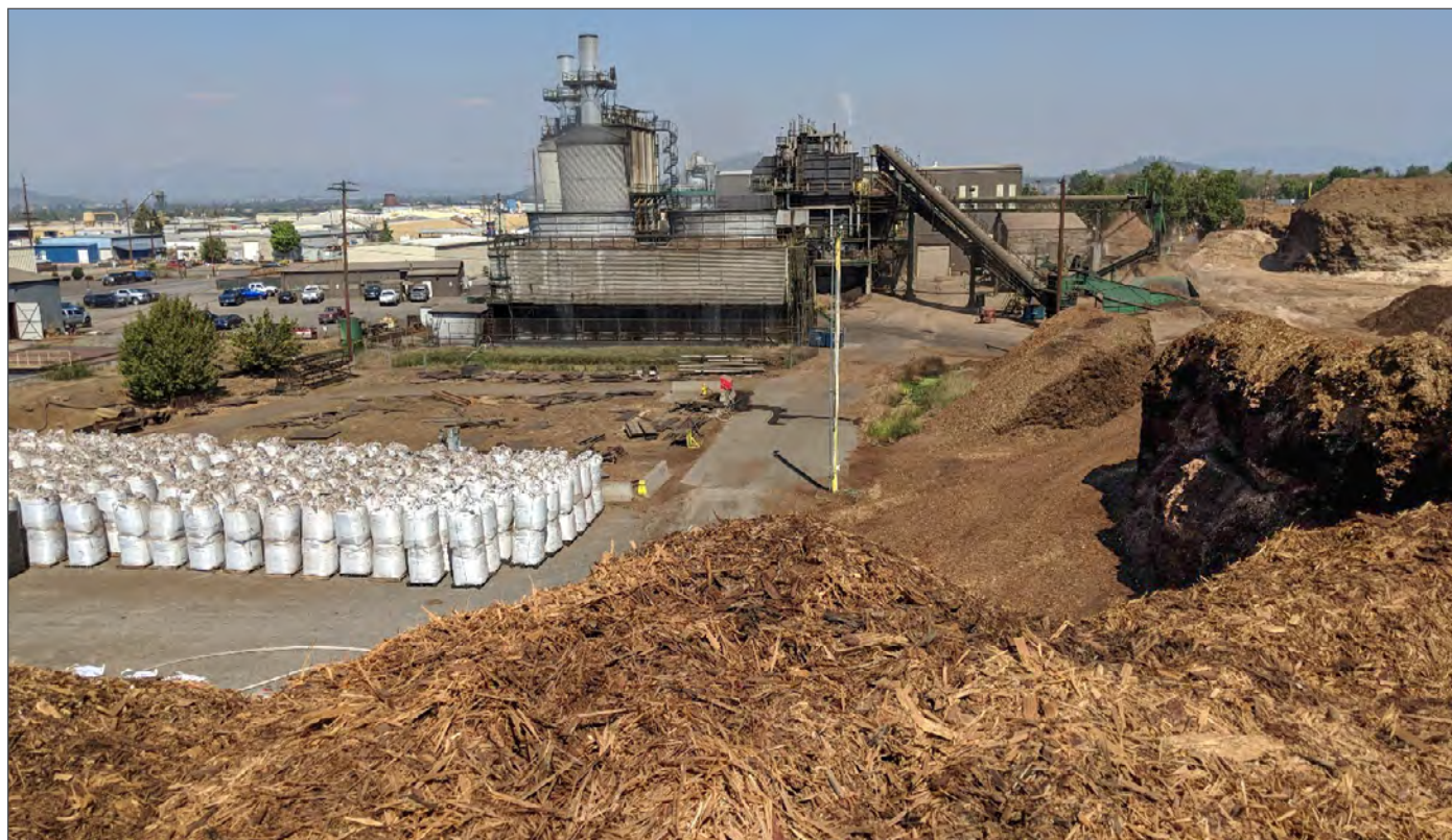
Figure 6.1. Biomass One in Medford, Oregon is an example of a centralized production facility. Production plant shown in background with hogfuel in foreground and supersacks of finished biochar. (Photo: Karl Strahl)
