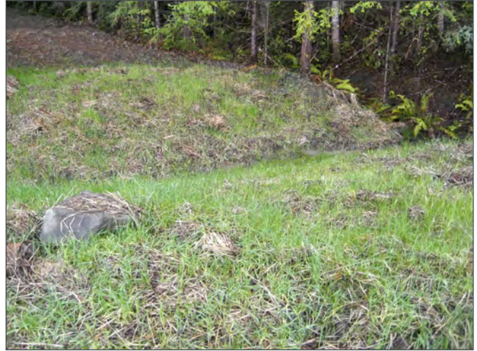
Figure 5.7. Forest road near Humboldt, California that has been decommissioned and revegetated to reduce soil erosion. (Photo: Han-Sup Han)
