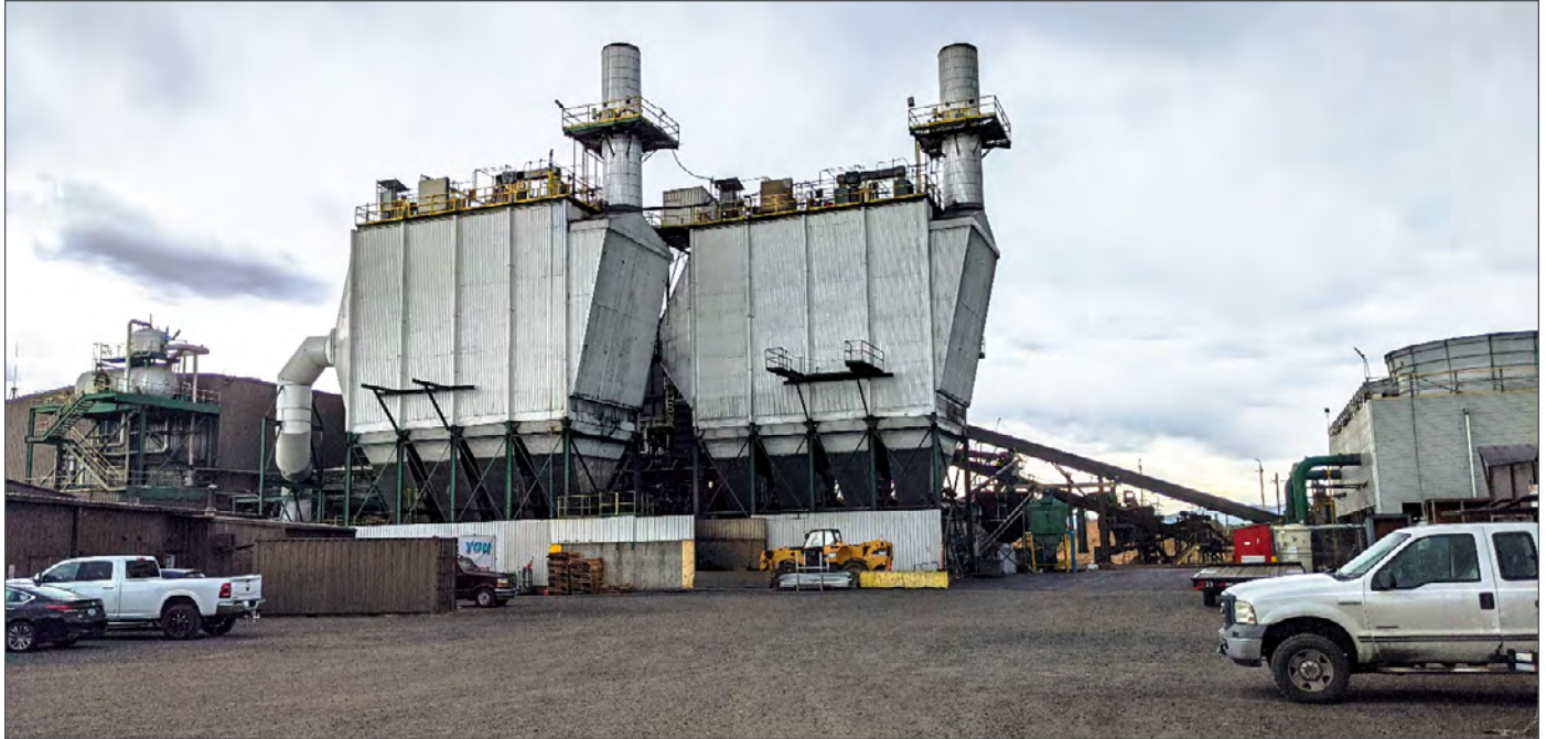
Figure 1.3. Biomass One in Medford, Oregon is a biomass power plant generating 32.5 megawatt electrical (MWe) (28.5 MWe goes to the grid). This plant consumes 200,000 tons per year of dry biomass and can recover 50,000 cubic yards of biochar annually (Photo: Karl Strahl)
