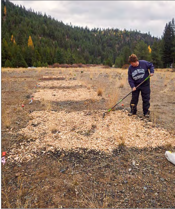
Figure 5.8. Installation of mine site restoration treatments on the Umatilla National Forest near a newly restored stream near the Granite Gold District which had been dredged for gold throughout the 19th and 20th centuries. The rock tailing piles near the stream were flattened and capped with silt loam in the 1970's, but little vegetation had developed. Treatments were wood chips, biochar, and biosolids. (Photo: USDA Forest Service)
