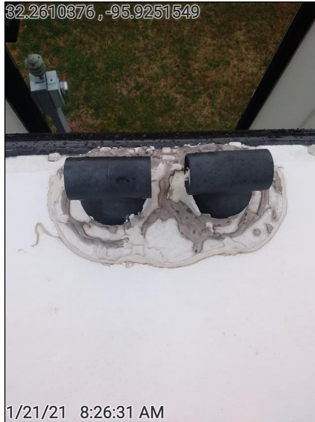
Plumbing vent cover.
