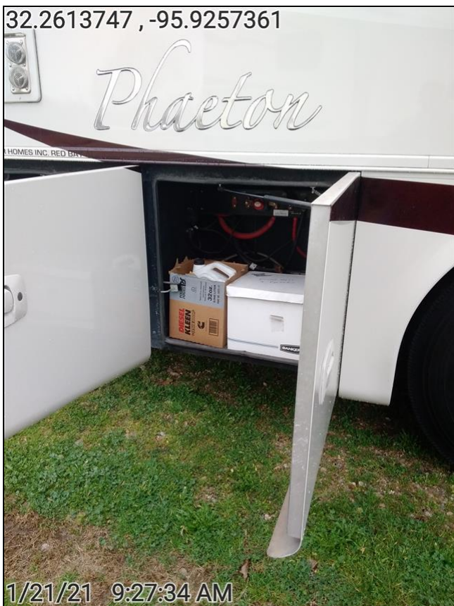
Chassis Battery compartment
