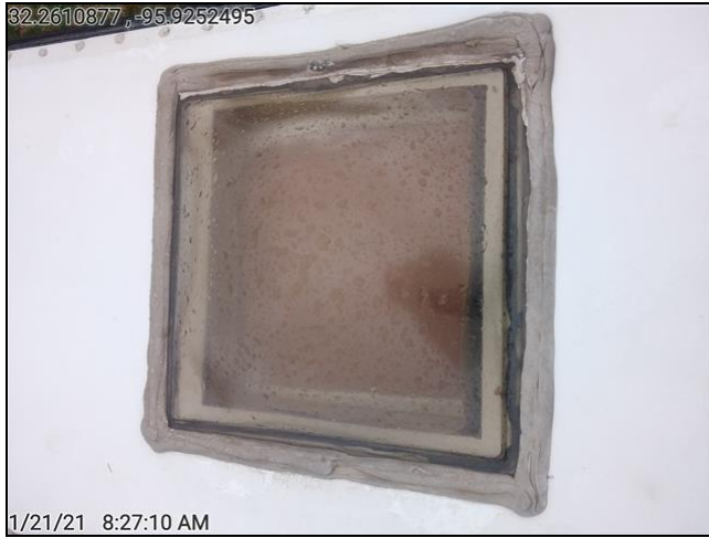
Main bath skylight
