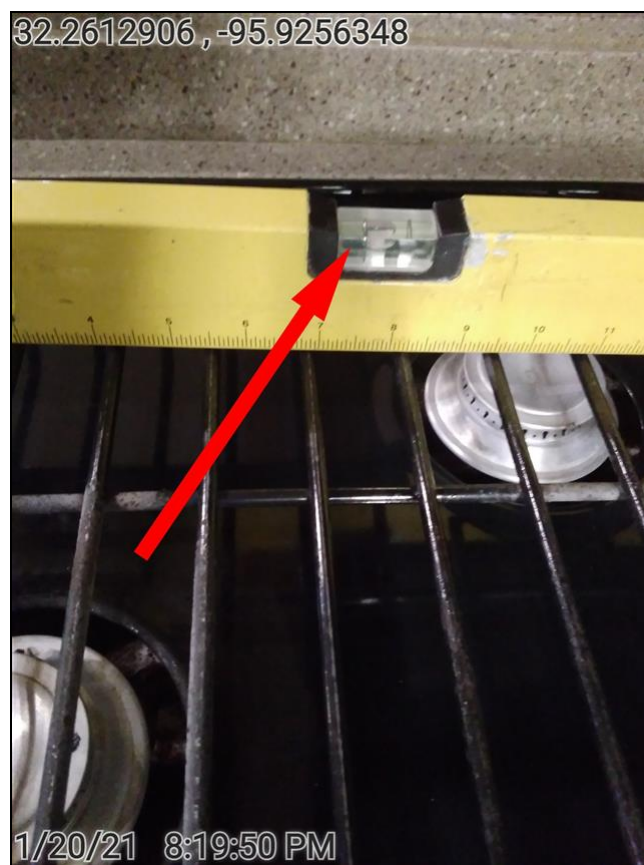
Stovetop out of level and high on drivers side.
