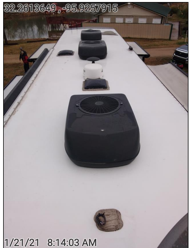
Roof facing rear
