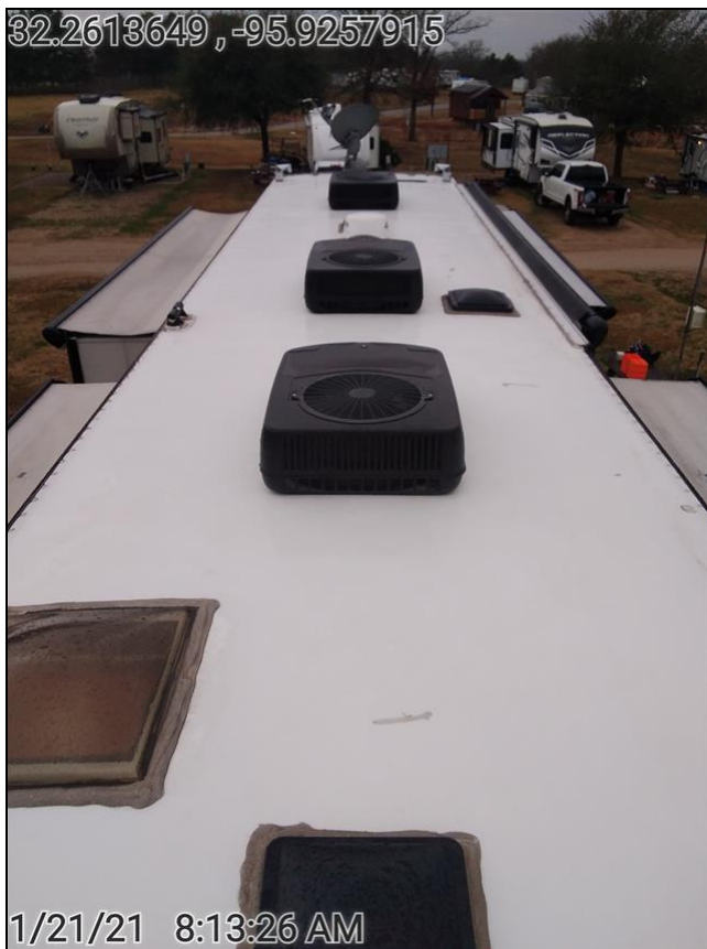
Roof facing front
