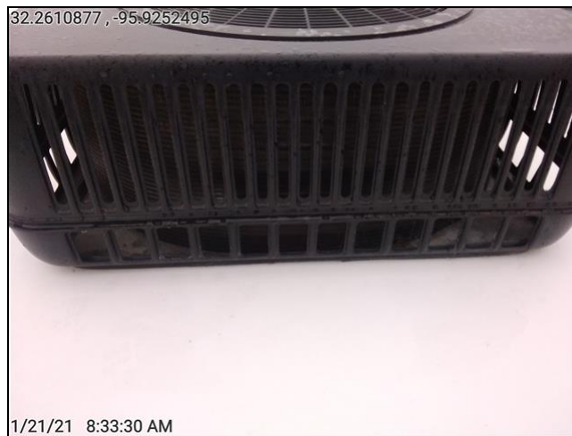
Rear AC coils.
