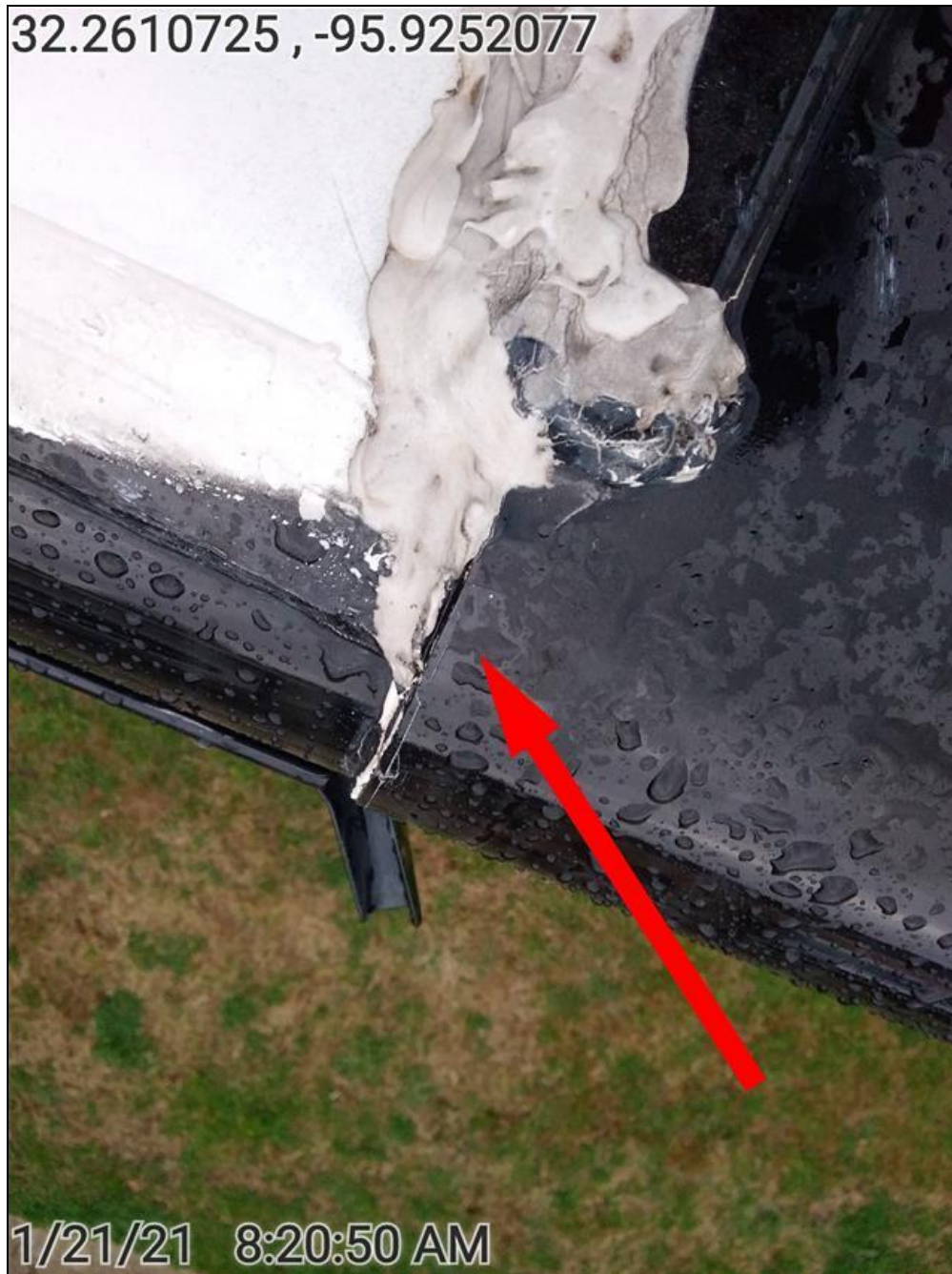
Streetside rear cap meets roof
