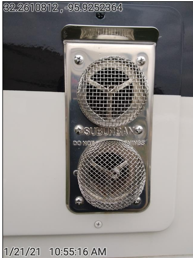
Furnace in the curbside front slide
