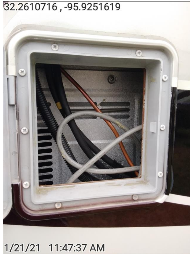
Refrigerator Rear Access
