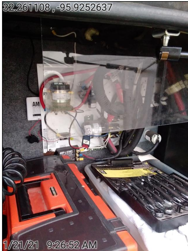
12 v control relays
