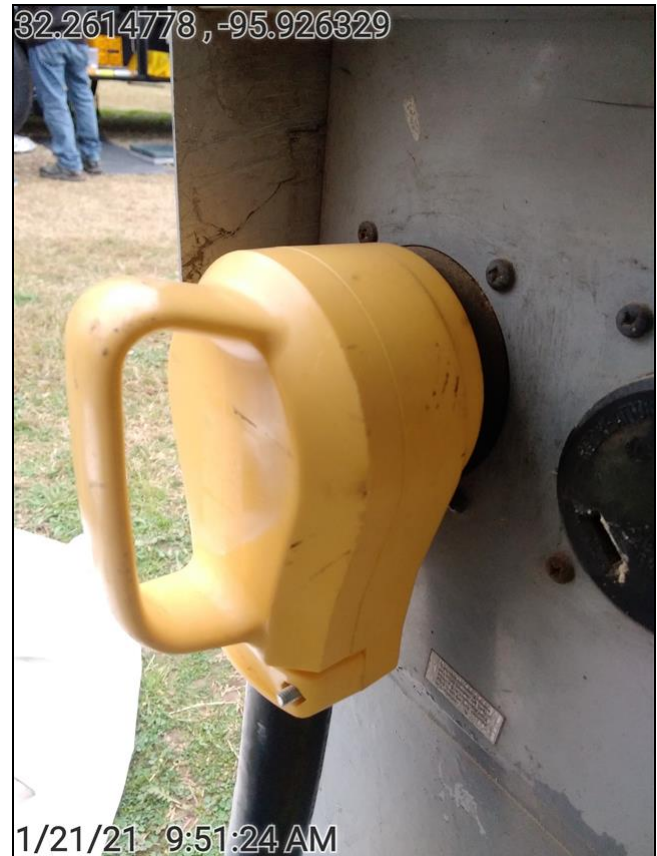
Shore power cord at pedestal
