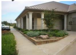
In this picture the bed was surrounded by low walls to provide better drainage on a level plane to prevent soils from washing over the sidewalks—it took 4 yards of enriched topsoil to raise the bed level approximately 4” in this 324 square foot bed—and 3” of mulch was added to that ( always allow for mulch when planning)
