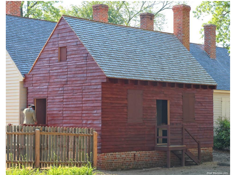
Exterior of the Anderson Armoury Tin Shop.
