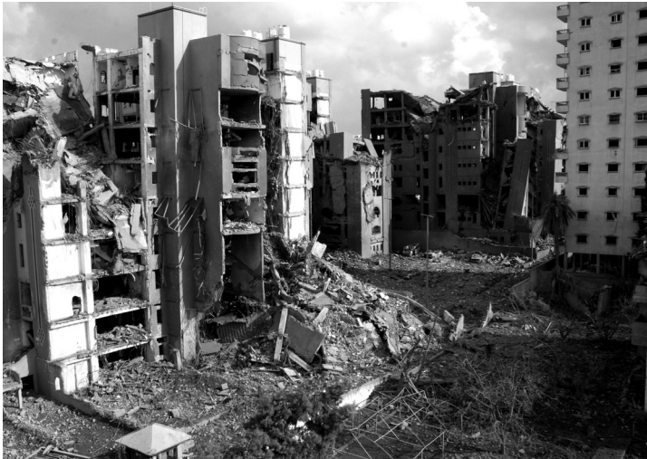
30th December 2008: Mojma Al-Wezarat, Tal El-Hawa, Gaza City. The ruins of bombed official government buildings (Mohammed Al-Zaanoun and Majdi Fathi)
