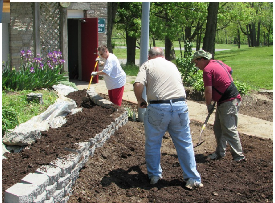
Members installing new soil at clubhouse May 2018
