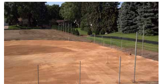
Above: field construction at Wilshire Park
