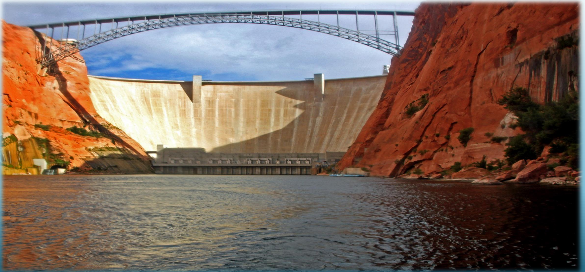
Glen Canyon Dam located in Page, AZ
