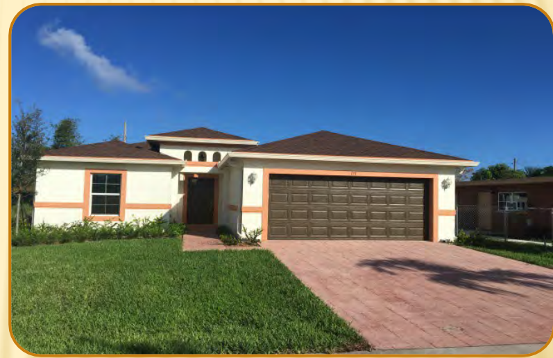
Work Force Housing Development
