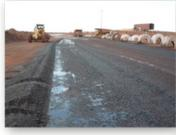
Apply the calculated volume of the dilute DCP30 solution to the area by means of multiple spray passes from the water bowser (truck). Multiple spray passes\* will ensure better penetration and will prevent product run-off.
