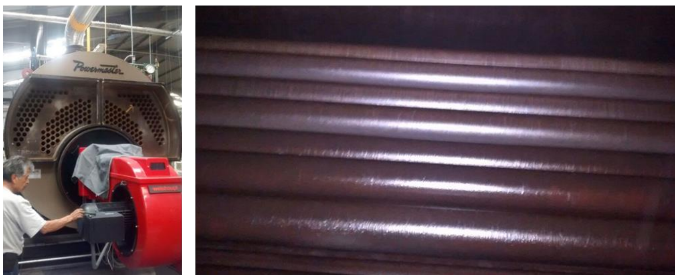
Figure 14: Inspection of 500 HP boiler, December 2015, after 6 months of tannin treatment.
