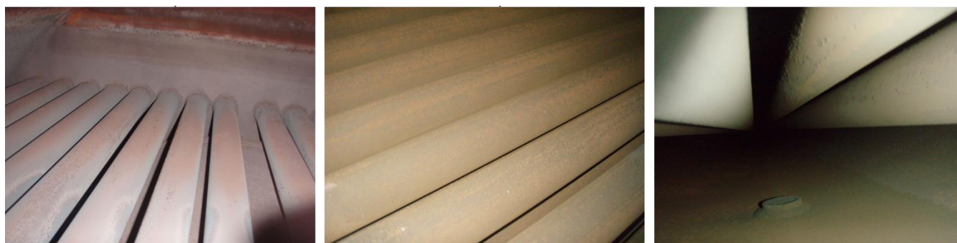
Figure 2: 2014 inspection of top (left and middle) and bottom (right) tubes while using conventional treatment.
