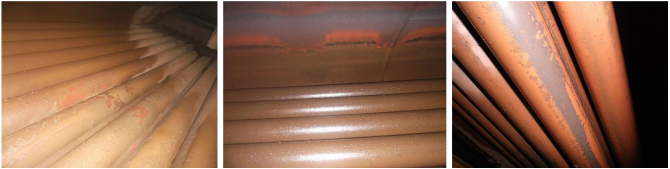
Figure 3: 2015 inspection of top (left and middle) and bottom tubes while using tannin treatment.
