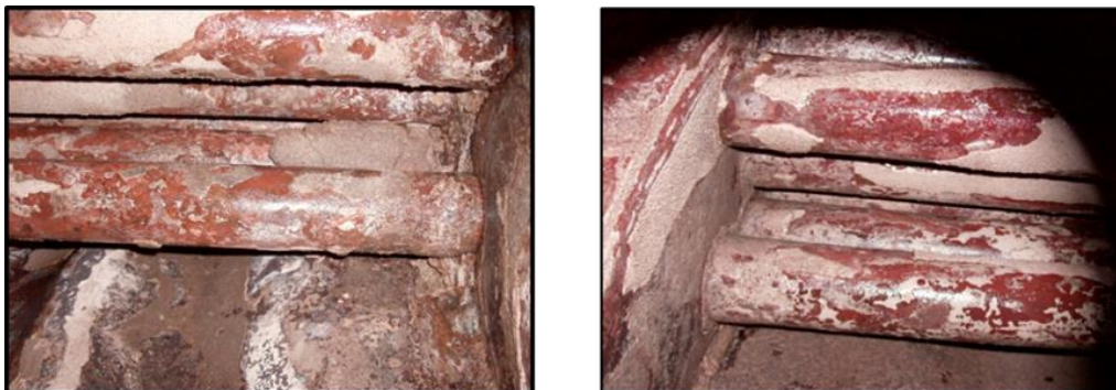
Figure 21: 2009 boiler tubes inspection after 4 months of Purified Tannin treatment.
