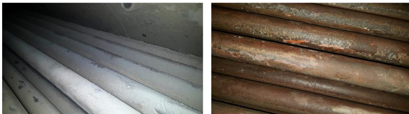
Figure 13: 200 HP boiler, December 2014, conventional treatment (left); June 2016, after one year of tannin treatment (right).
