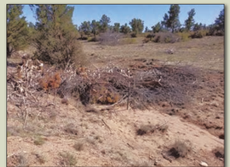
Juniper silt dam installed for erosion control. Photo Credit: UVRWPC
