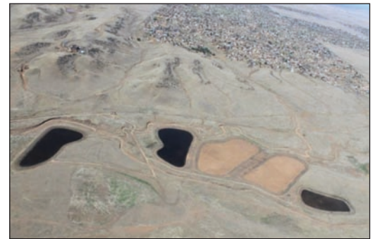
Aerial view of recharge basins located west of Prescott Valley.
