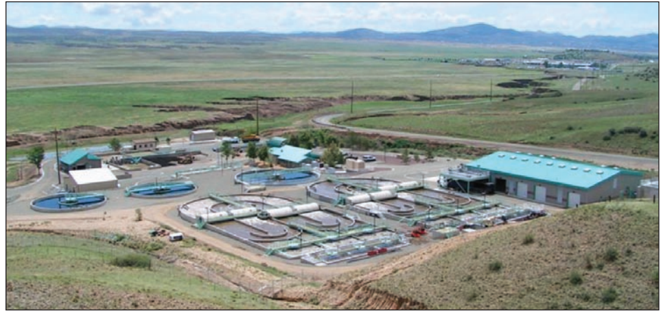
Town of Prescott Valley Advanced Treatment Facility
