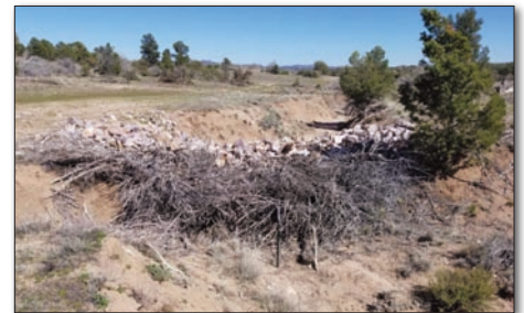
View of juniper silt dam installed on the Barney-York Ranch
