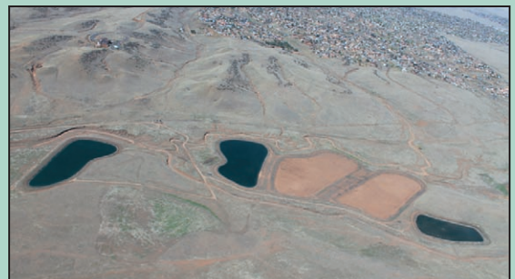
Town of Prescott Valley recharge facility
