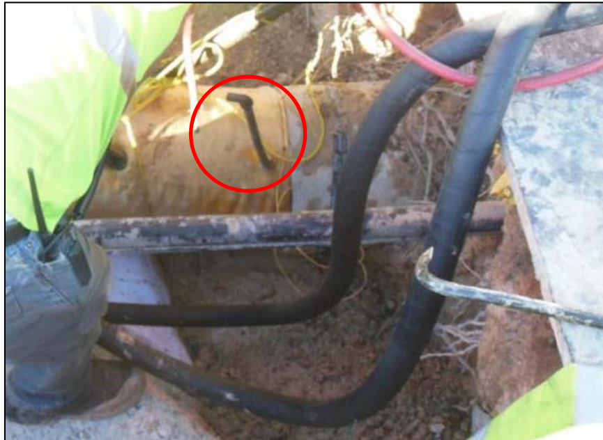
Figure 4-15 Condensation vent extending from the liner at Station B
