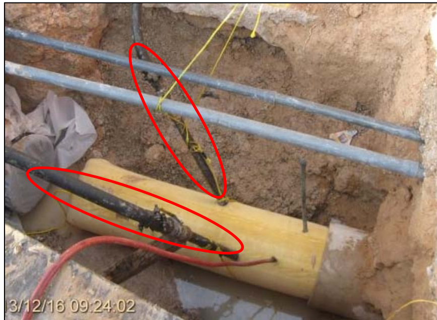
Figure 4-11 End of liner with stingers at Station B
