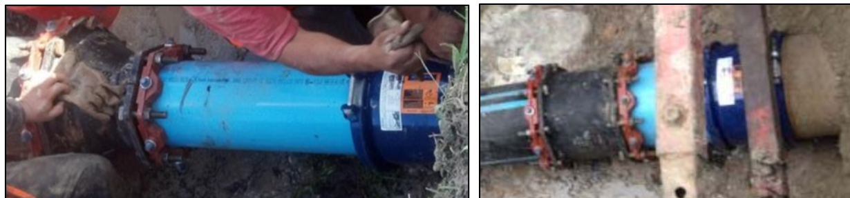
Figure 3-16 Connection between HDPE and AC with reducer (left) and sleeve (right)
