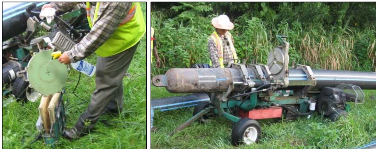
Figure 3-4 Flat iron with heating element (left) and pipe fuser (right)
