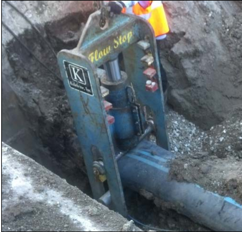
Figure 3-11 Hydraulic pipe clamp
