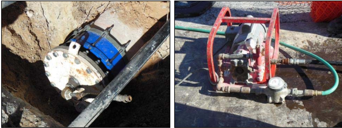
Figure 4-23 End cap with garden hose connection (left) and small electric pump (right)
