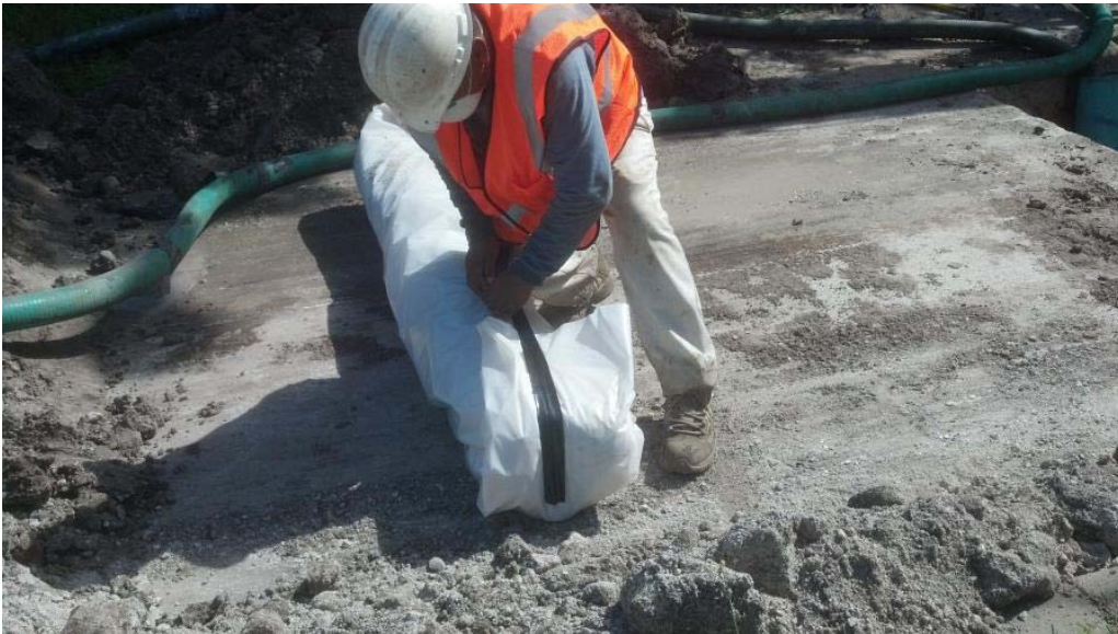
Figure 2-2 AC pipe being wrapped in plastic for disposal
