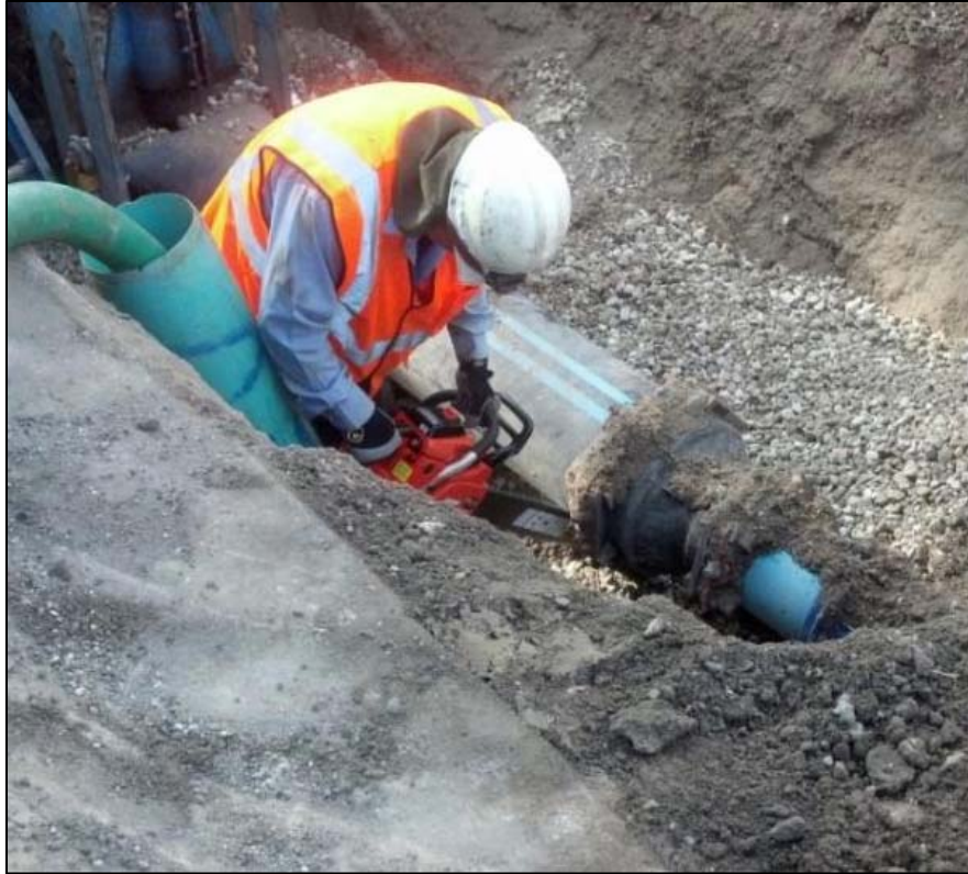
Figure 3-12. Removal of temporary connection
