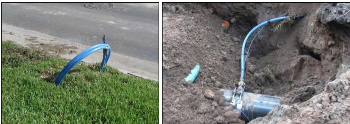
Figure 3-3 New HDPE service (left) and service connected to new HDPE main (right)
