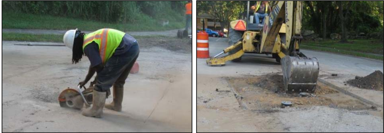
Figure 3-6 Pavement cutting (left) and pit excavation (right)
