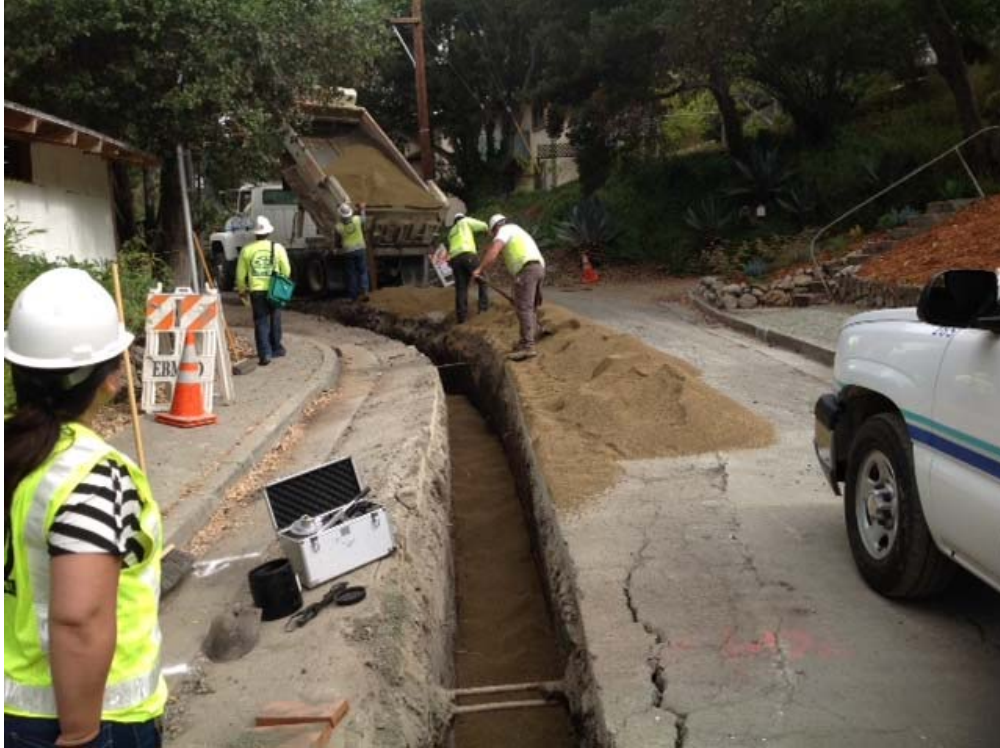
Figure 2-1 Typical open cut installation site
