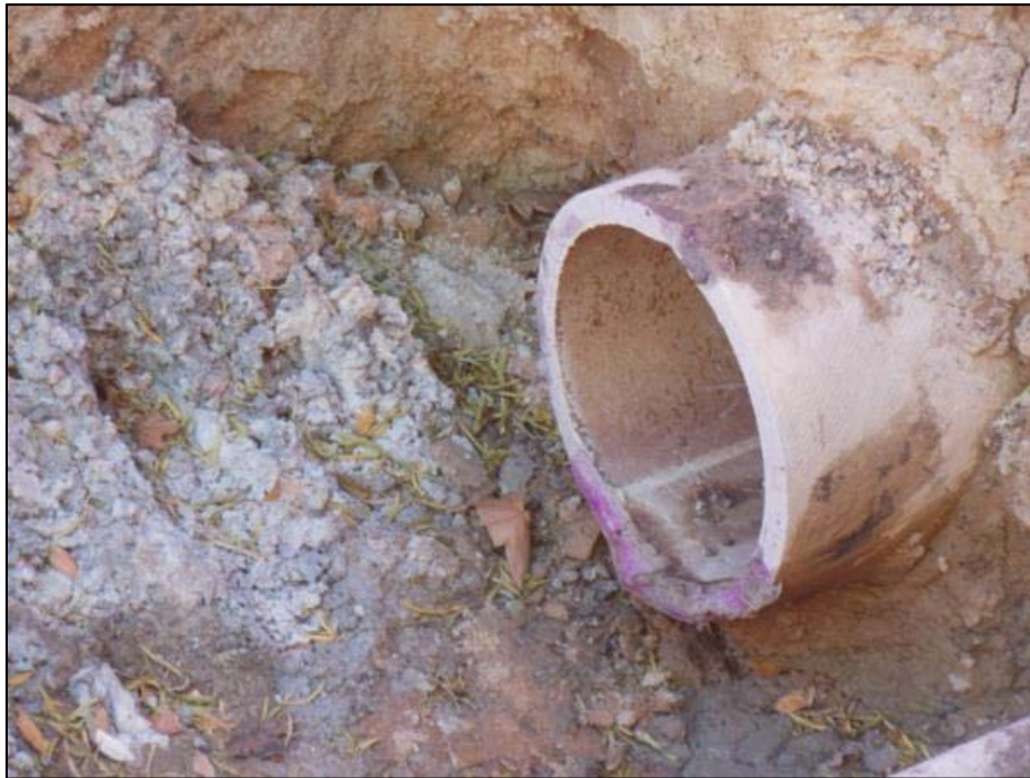
Figure 4-3 Cut AC pipe protruding from the pit wall
