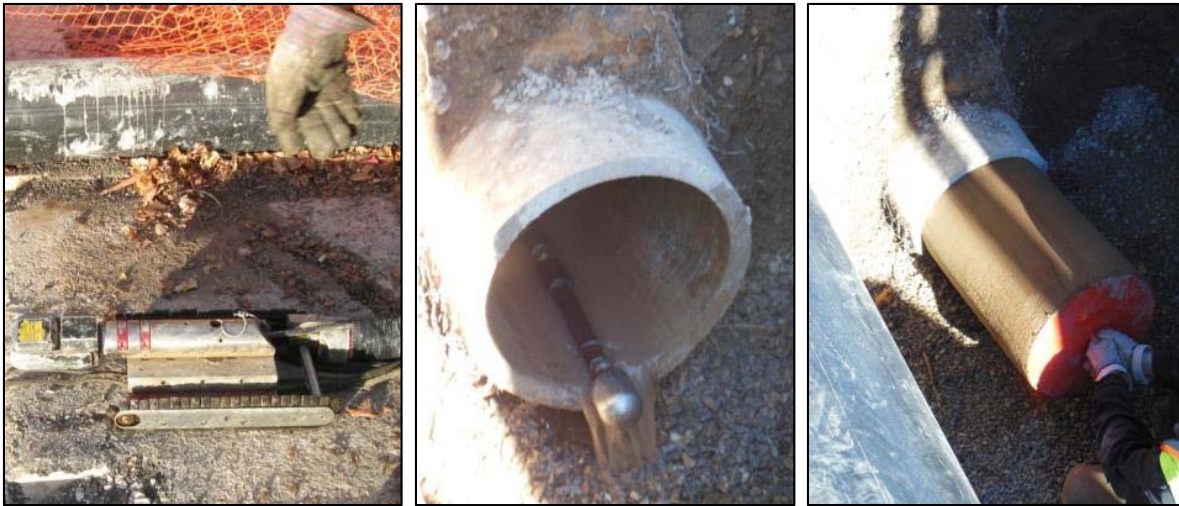
Figure 4-4 Equipment: camera (left), water jet (center), and squeegee (right)
