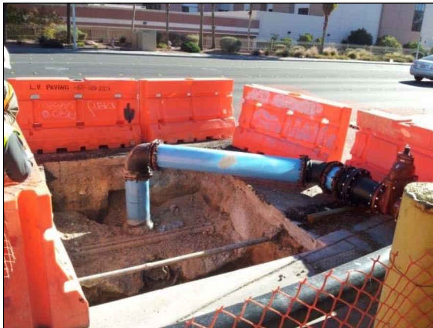
Figure 4-1 Access pit along roadway barricaded and fenced off
