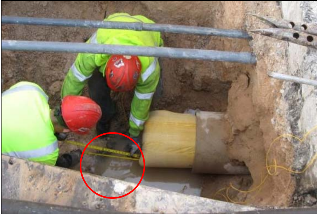
Figure 4-9 End of liner with rope arriving at Station B
