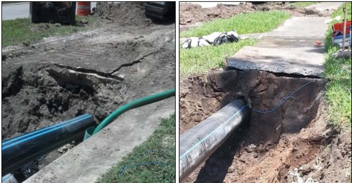
Figure 3-15 Upheaval of roadways and sidewalks during runs #2 (left) and #6 (right)
