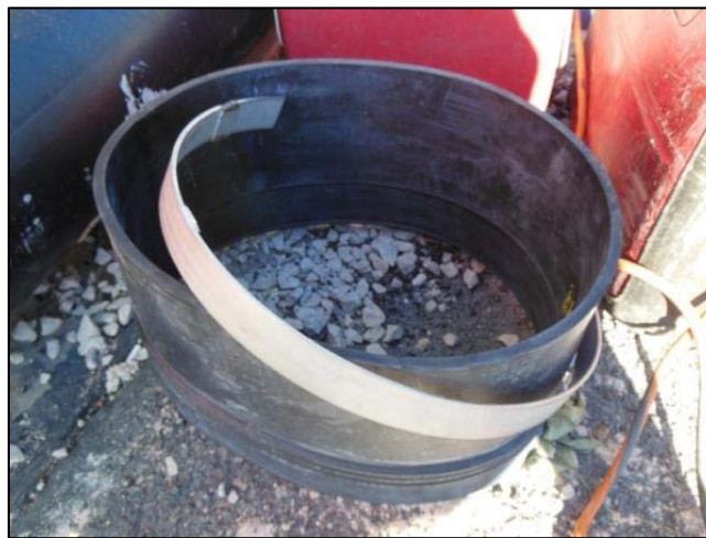
Figure 4-17 End seal consists of a rubber gasket and steel rings
