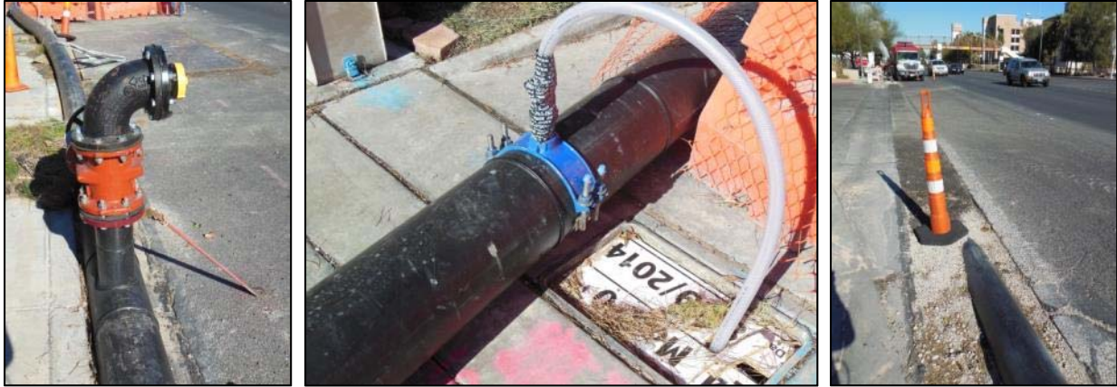
Figure 4-2 Bypass system: hydrant (left), service (center), and buried entrance (right)
