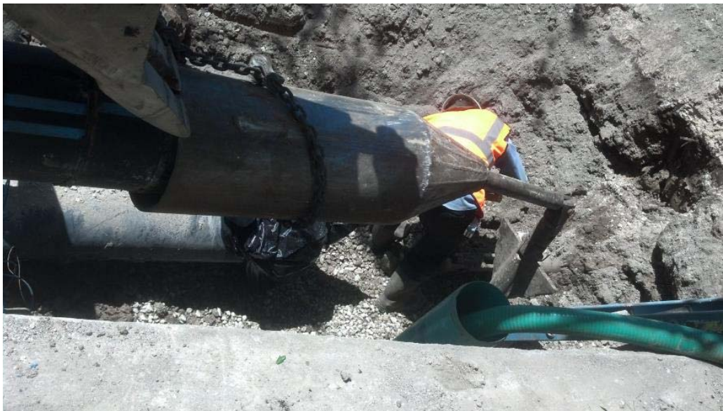
Figure 2-5 Pipe bursting used to renew an 8-in AC water main
