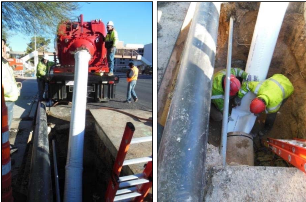
Figure 4-8 Protective sleeve and pressure vessel (left) and guiding the liner in (right)
