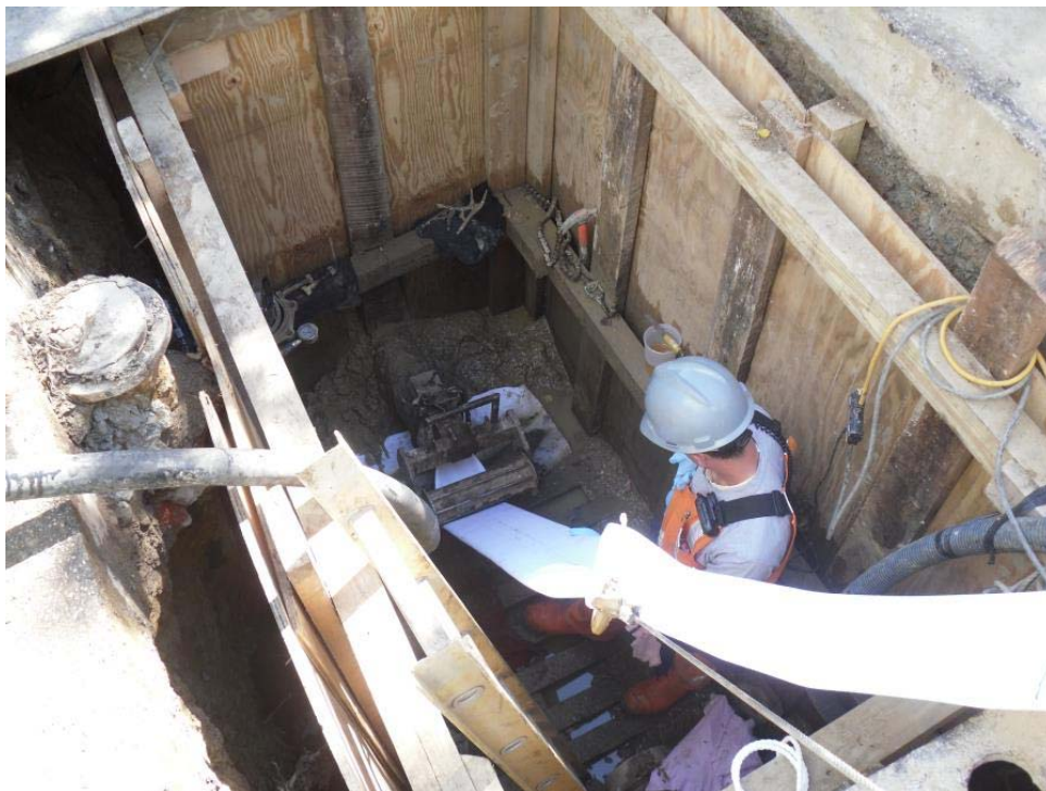
Figure 2-3 CIPP used to renew a 6-in water main
