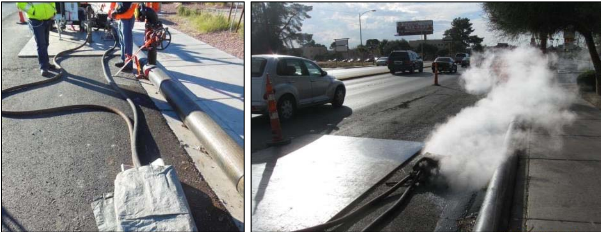
Figure 4-13 Hoses used to vent steam during the curing process
