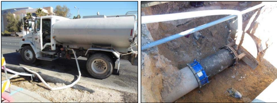
Figure 4-22 Truck pumping water in the pipe through an end cap for a pressure test
