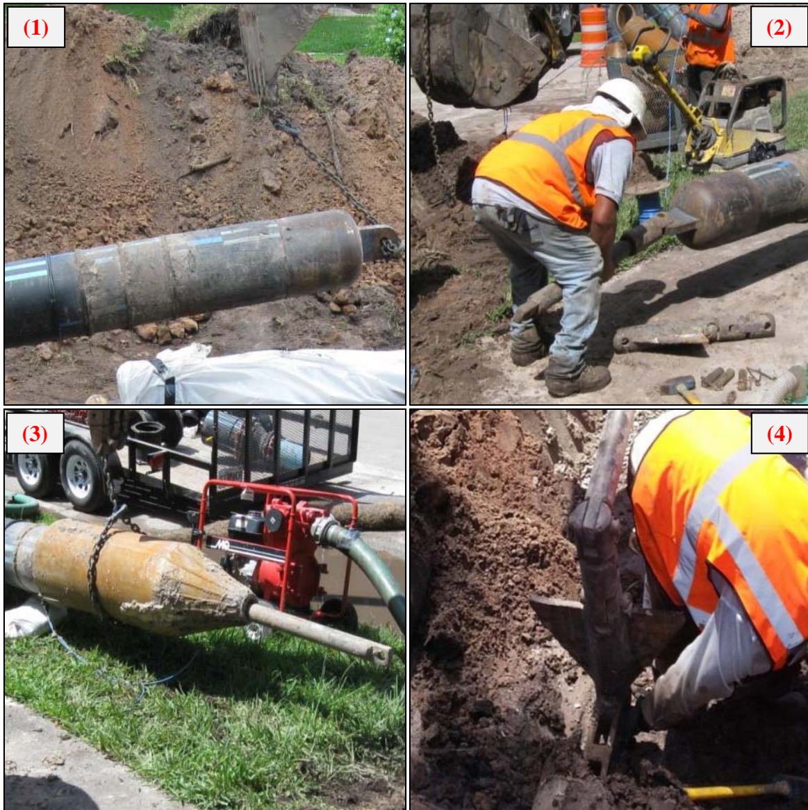
Figure 3-13 Elements of the bursting head
