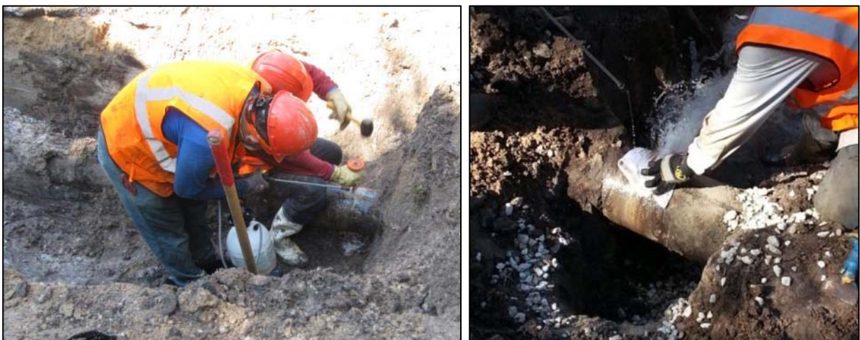
Figure 3-7 Workers cutting AC pipe
