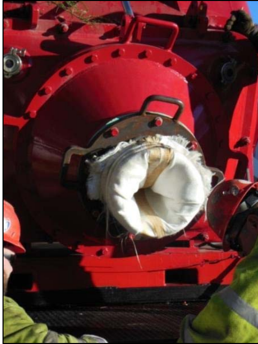
Figure 4-7 Inverted liner end attached to pressure vessel opening
