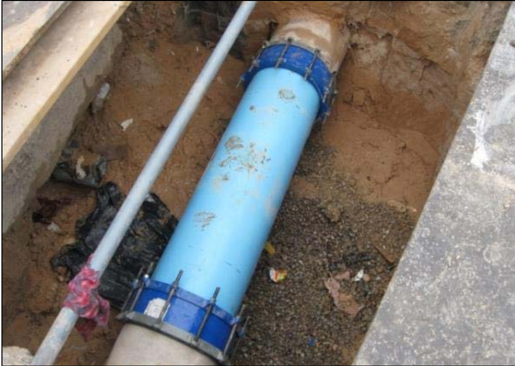
Figure 4-24 Lined AC pipe sections connected by a 16-inch PVC pipe
