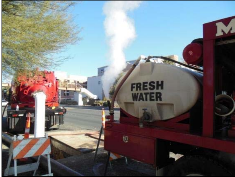
Figure 4-10 Steam truck (foreground) connected to inversion truck (background)
