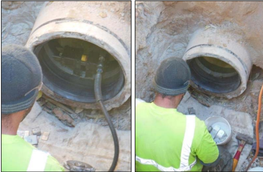
Figure 4-18 Hydraulic ring opener (left) and finished inner ring on end seal (right)
