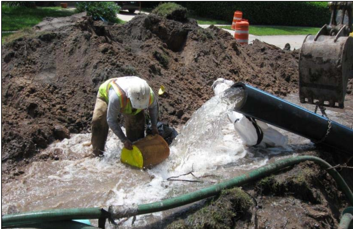
Figure 3-18 Cleaning of HDPE pipe using super-chlorinated water and polyswab
