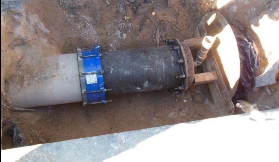
Figure 4-21 End cap assembly connected to AC pipe for a pressure test
