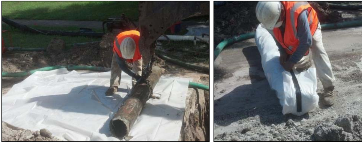
Figure 3-8 Wrapping and taping of the AC pipe
