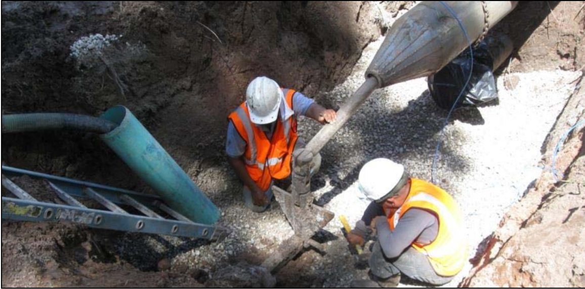
Figure 3-14 Fully-assembled bursting head connected to linkage at insertion pit
