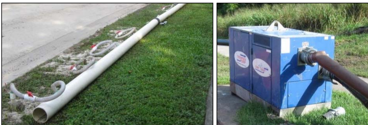
Figure 3-2 Dewatering system (left) and pump (right)
