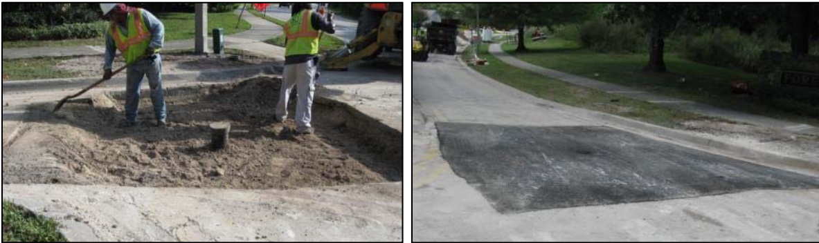
Figure 3-20 Preparation and repaving of pit #1 by restoration crew
