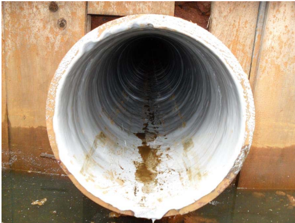
Figure 2-4 SIPP used to renew a 10-in water main
