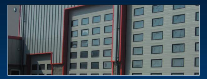
Overhead doors are selected for their high levels of thermal performance as well as noise reducing properties which make them ideal for factories or warehouses. Their rigid construction makes them a reliable option in high-usage applications.
