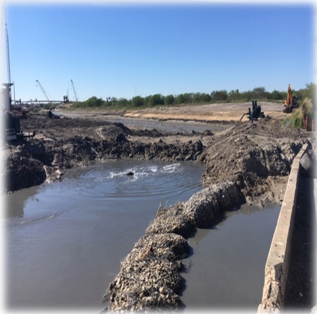
Rock filter dam limiting sedimentation into the Salt Flat Channel, and downstream to the Ship Channel
