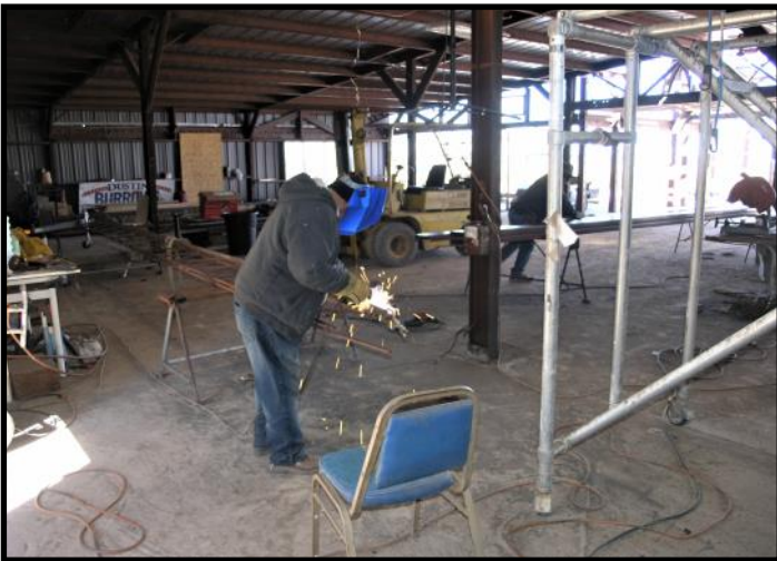
Sparks fly as Manuel Constancio works on the ceiling beam. The area behind him will be the new conference room.
