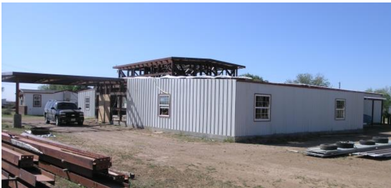
The siding on the lower section of the building is almost complete.
