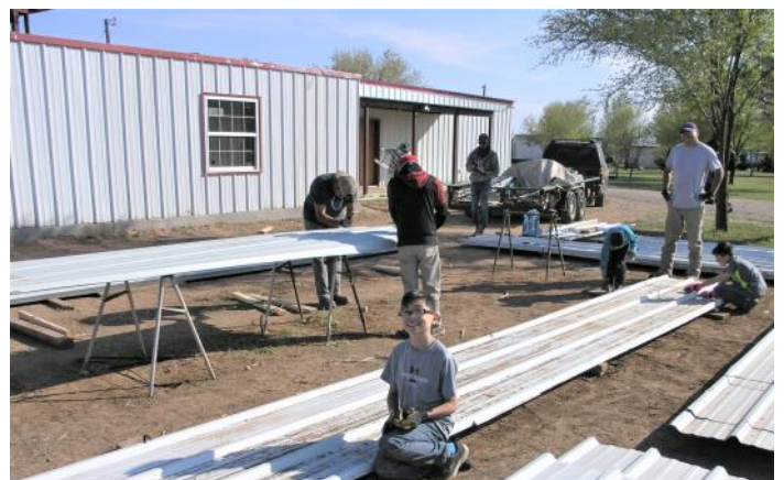
Ralph Mendez and his sons help clean up the panels for the new roof.
