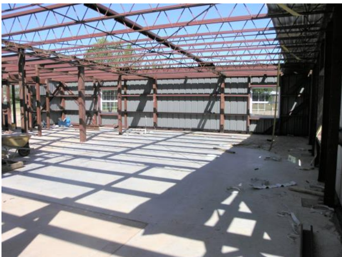
The gift shop waits for the installation of the roof.
