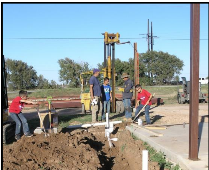
Isidore Martinez, Ralph Mendez along with sons are finishing up the plumbing for the Rest Rooms that will be located next to the new Gift Shop. Ralph's sons can be seen filling in the ditch to cover the plumbing. Go to WWW.flameofmercy.com to see more pictures and current on construction.
