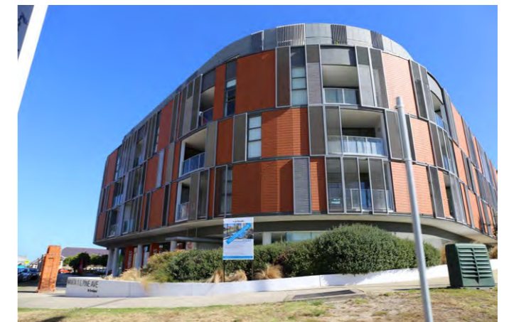
6. Four storey apartment building with ground floor retail
