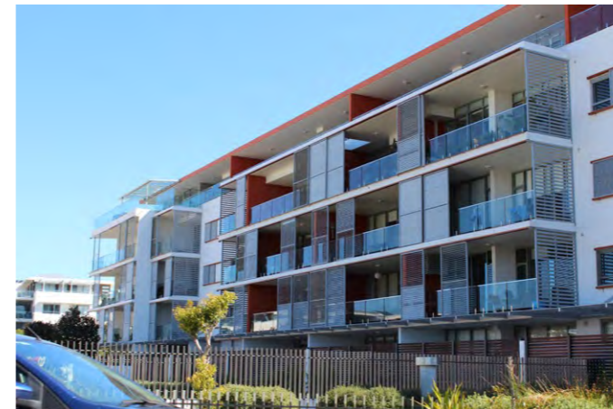
5. Five storey apartment building to the south
