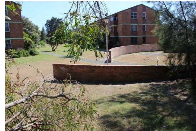
2. Three storey walk up public housing to the north
