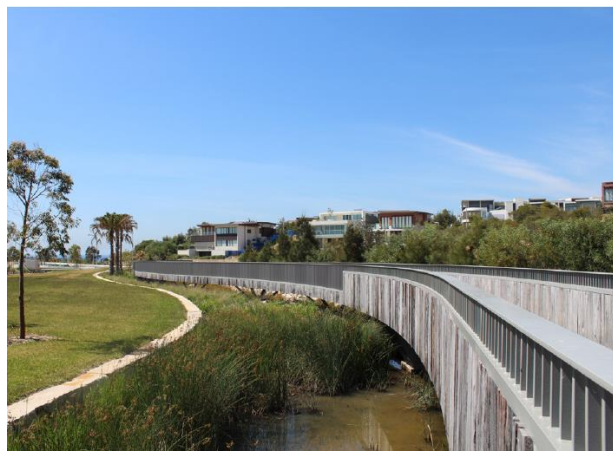
Figure 7 – Existing footbridge currently on the site
