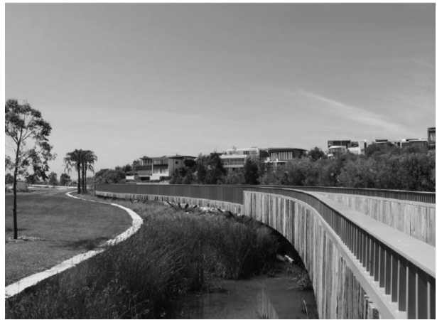
Picture 4 – Existing footbridge currently on the site
