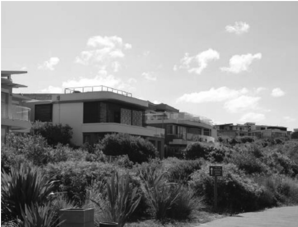
Picture 7 – Neighbouring development to the south fronting golf course
