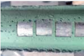
• Power Transmission Pipe Cleaning
