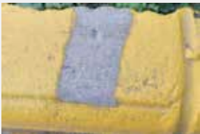
• Road Surface Paint Removal
