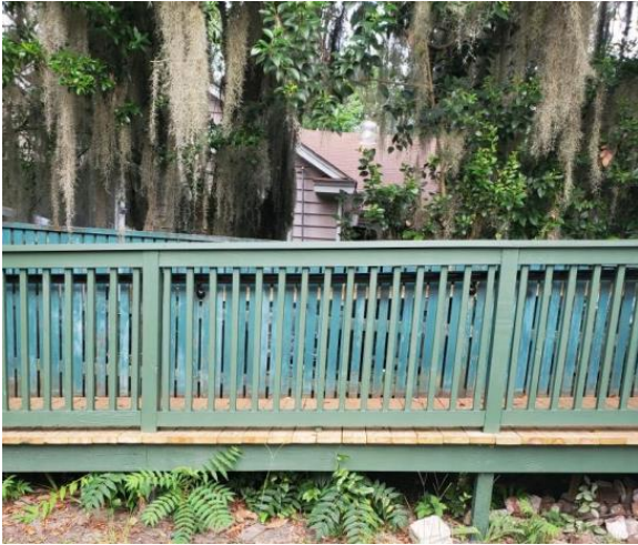
The restored accessibility ramp.
