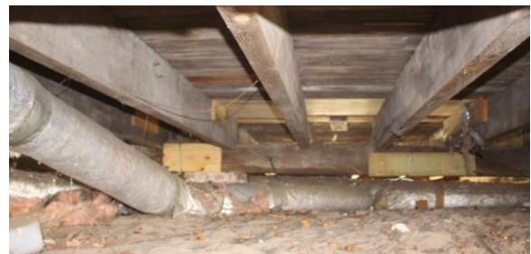
Repairs in the crawl space
