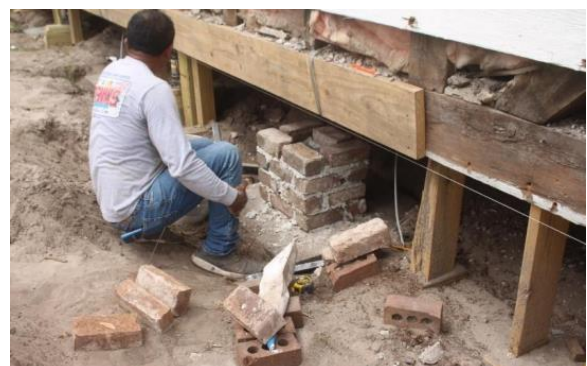
Rebuilding a foundation pier.
