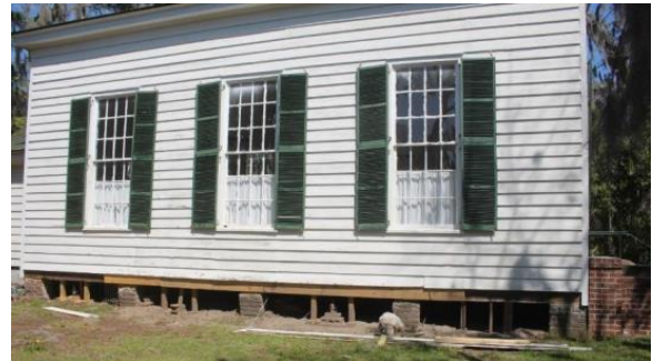
Side view showing the extent of the work.
