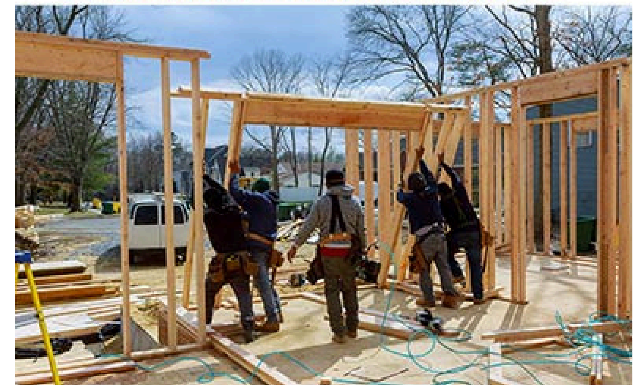
Stick Frame Construction Site
