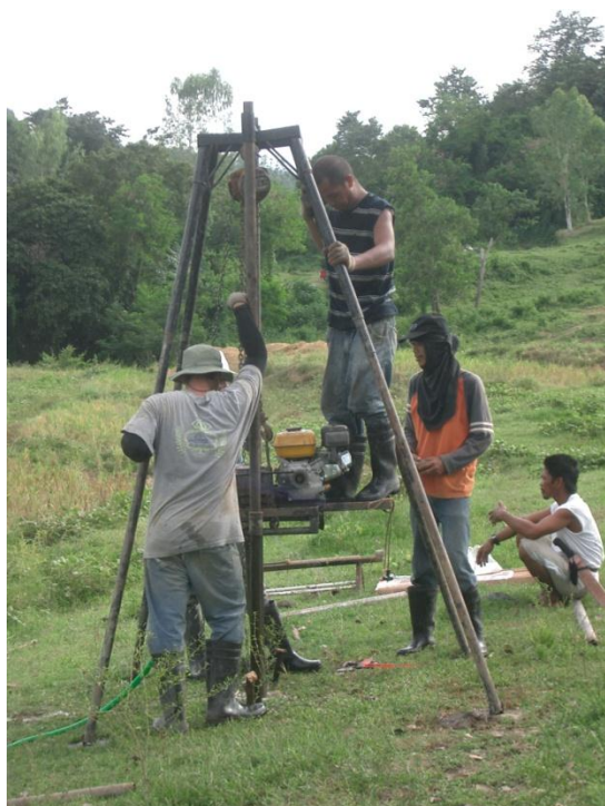
Figure 21: small diameter drilling machine on-site at Bigbiga. Borehole DH01, left and borehole DH04, right
