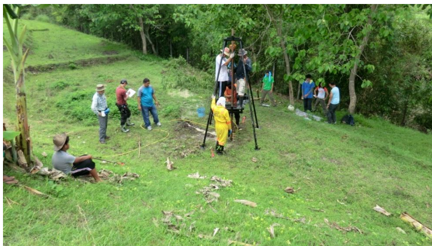
Figure 28: UP drilling rig and team drilling borehole DH05
