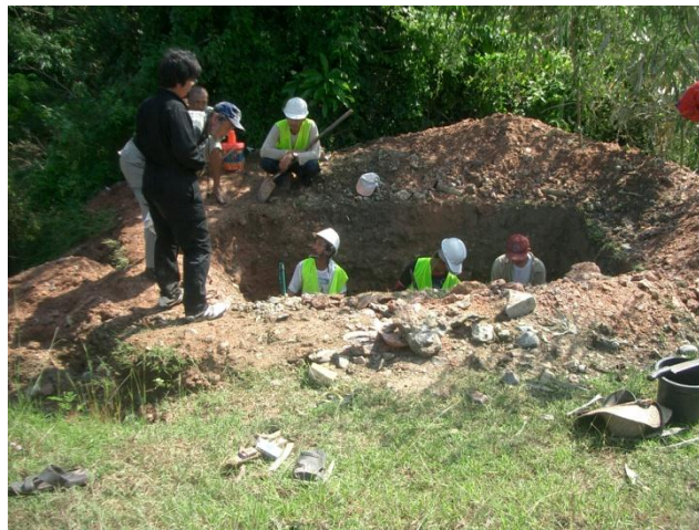
Figure 24: Trench BBT01 on west side of the Akrotiro River (see Figure 17 for the position) being excavated by hand
