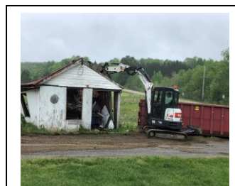
We removed an old building for additional parking at the market.
