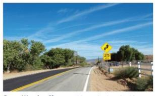
**Curve Warning Signs** provide emphasis and guidance for a change in horizontal alignment. Advisory speed signs may be used to supplement warning signs.
