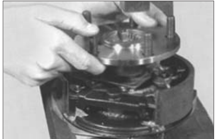
Figure 6-31. Bearing Supported In Press
