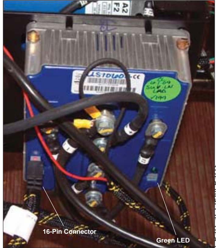
Figure 4-1. Controller Located Under Rear Seat or Utility Bed
