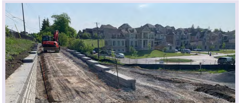
Pedestrian Trail Connection Derry Road West to Culham Trail
